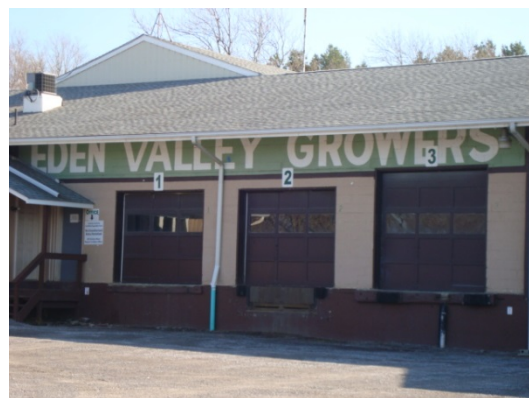
Figure 3. Loading dock at Eden Valley Growers
